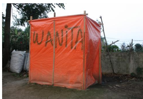
Photograph 4. Temporary Toilets in UKA Kabanjahe 1
