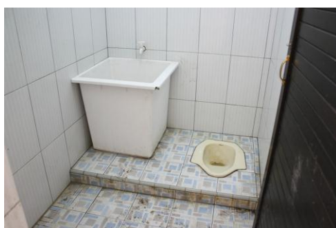
Photograph 3. Permanent Toilet Facility in Church (Klasis GBKP Kabanjahe)
